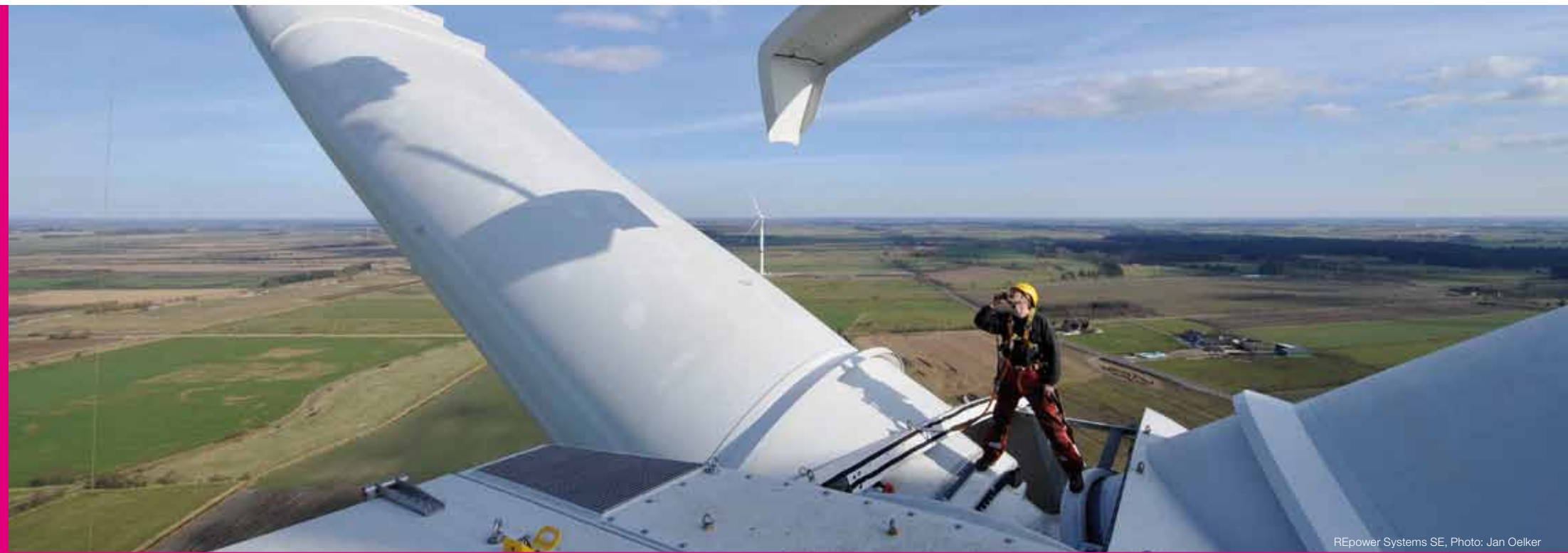
REpower Systems SE, Photo: Jan Oelker
